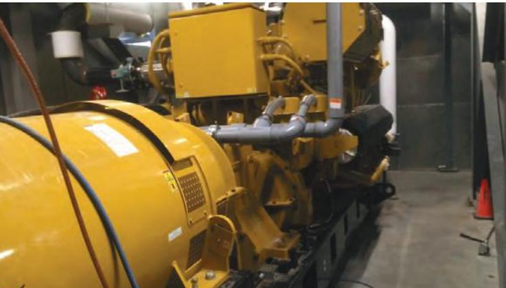
Figure 2: The Cogen Engine<sup>[5]</sup>
